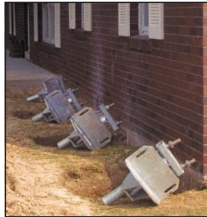
Anchor shafts are cut off, then brackets are attached.
