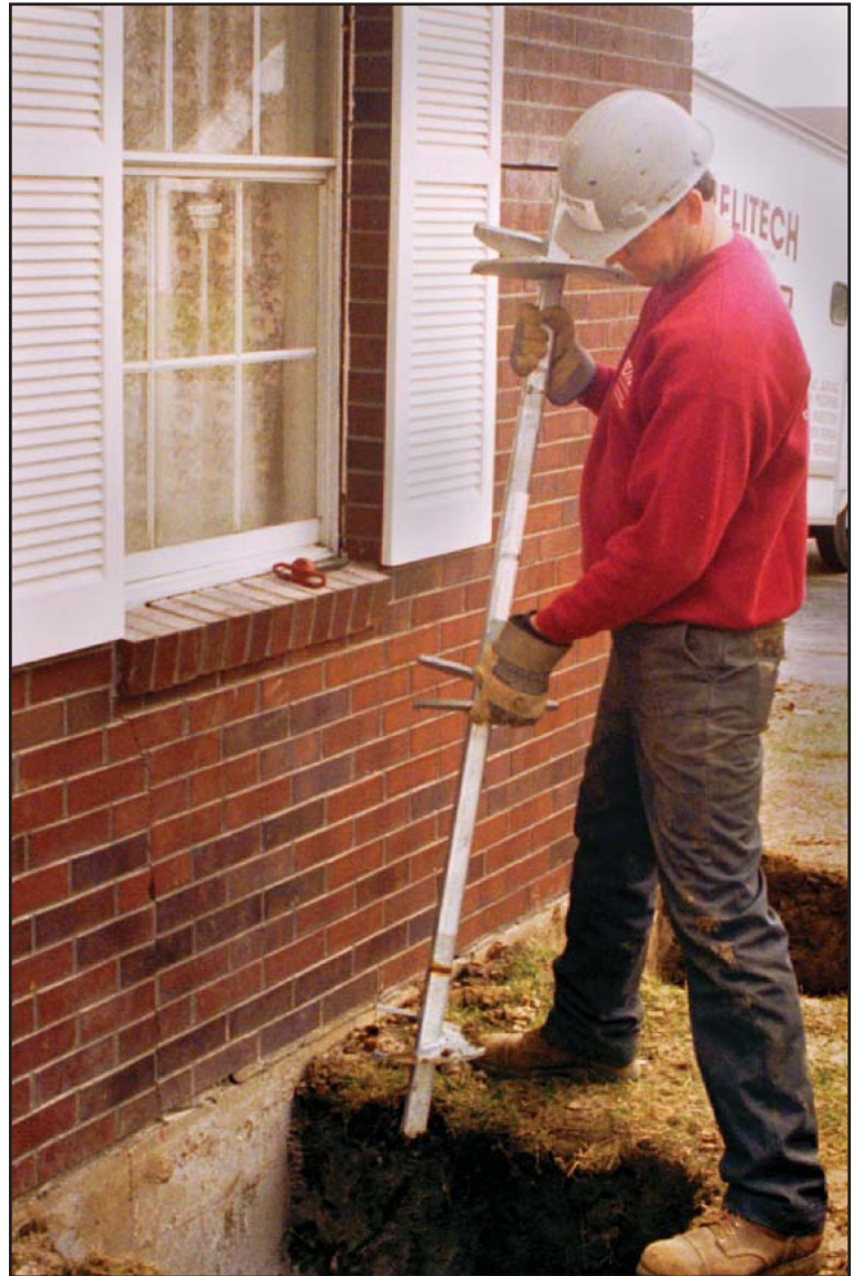
Placing a twin-helix anchor
